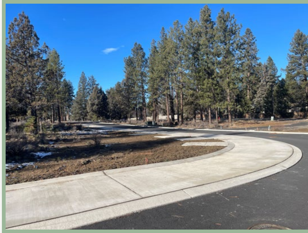
Alley Way with Concrete Parking Strip
