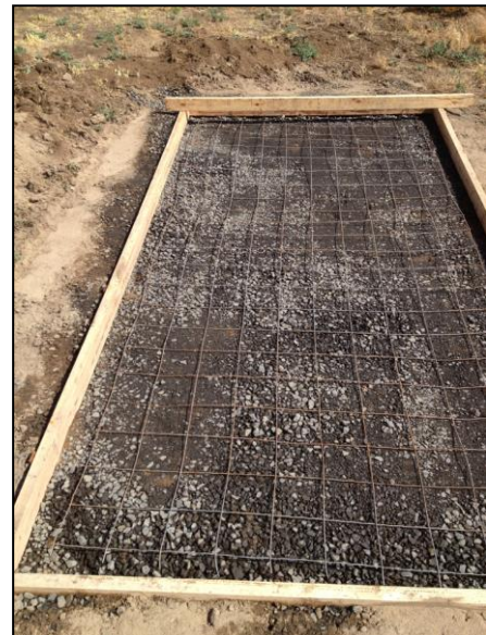
Wire mesh added for re-enforcement
